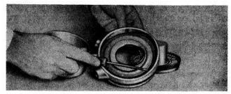
D. Remove the rubber washer and "0" ring from the Fail-Safe unit (use small screwdriver or other pointed tool).
